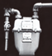
Meter Bypassing
