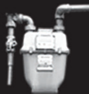
Meter Bypassing
