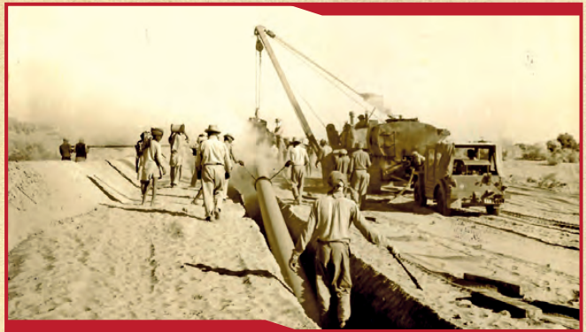
A pipeline lowering job in progress by the workers of SGTC during a project carried out in 1955 in Sindh
