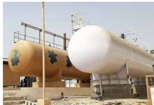
Against all odds: SSGC carried out a challenging task of installing LPG-Air Mix Plants in Awaran and Bela
