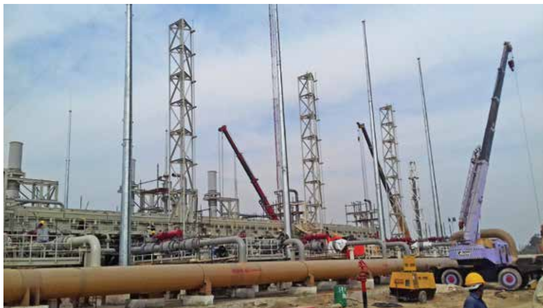
Aiming Higher: A view of HQ-2 facility in Daur near Nawabshah where the Company commissioned six compressors as part of the RLNG transmission project
