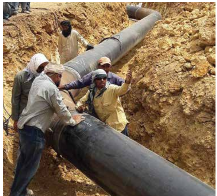
Winding paths: A pipeline construction activity in progress
