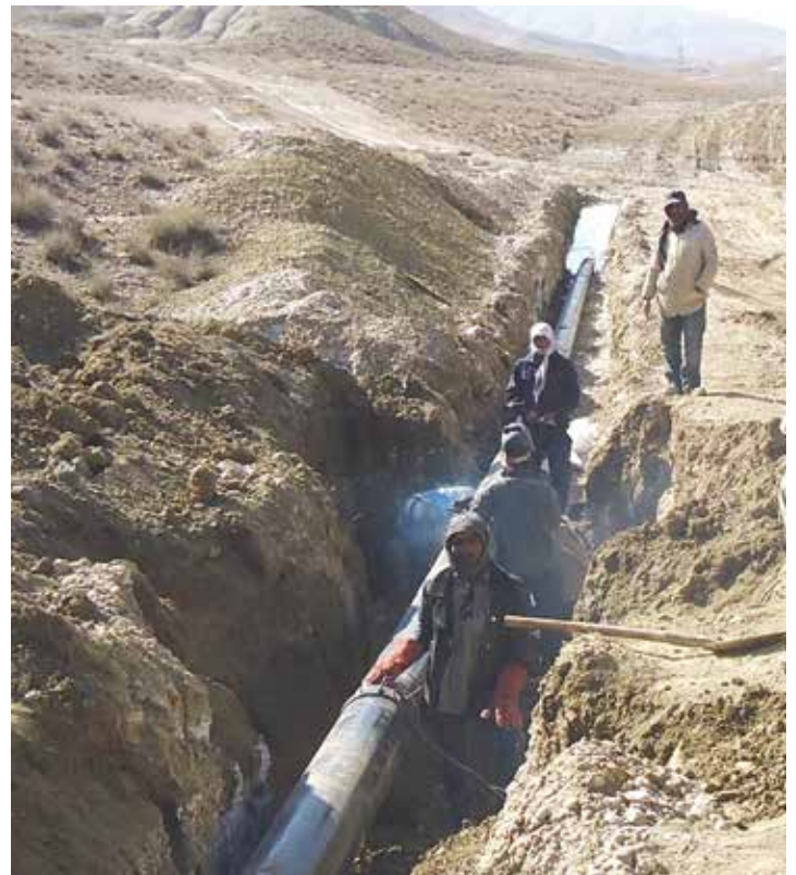
Through rough terrains: Pipeline laying activity in progress in Balochistan
