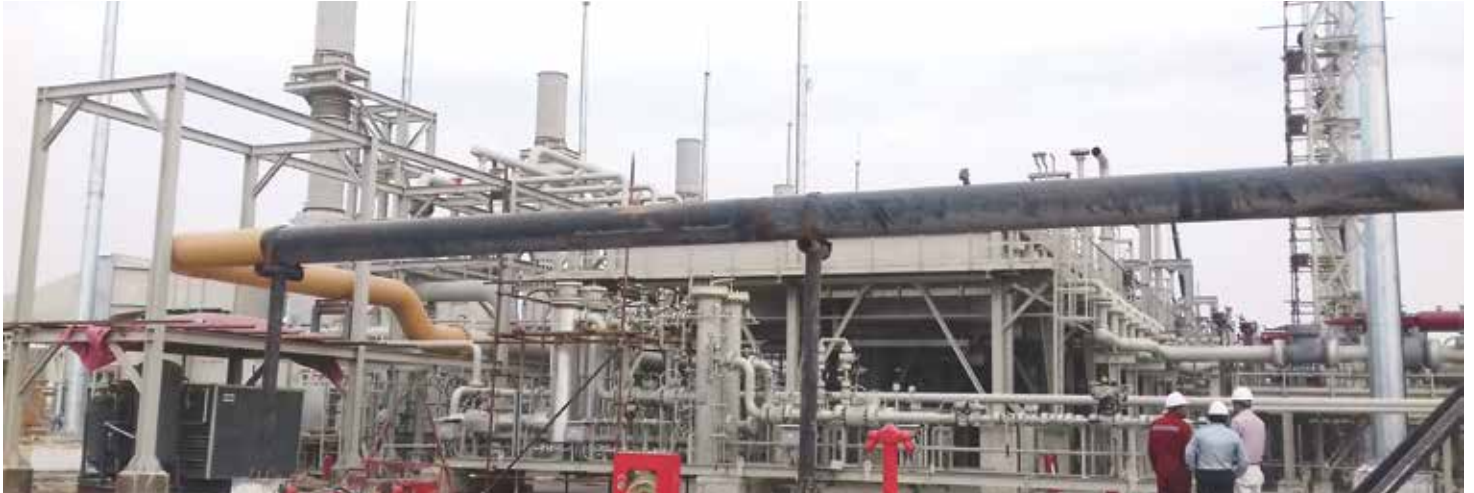
For achieving desired pressure: Installation of compressors in progress at HQ-2 Daur
