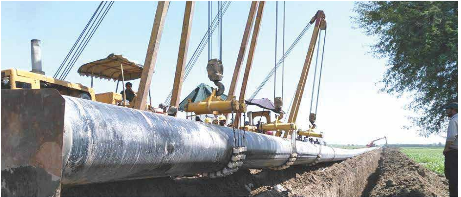
Total Commitment: Work on RLNG project in full swing in Lower Sindh
