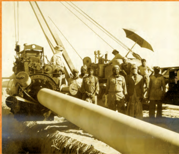
SGTC workers at the pipeline laying site
