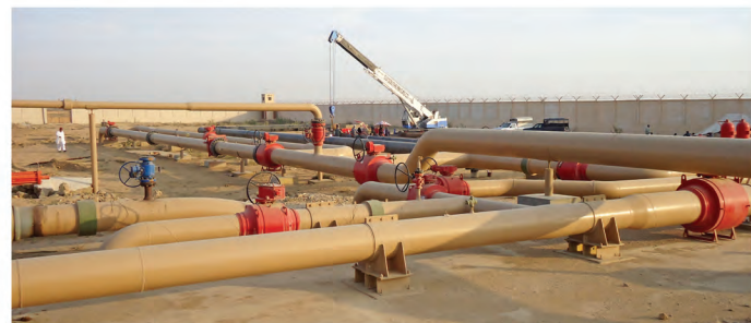
LNG work in progress at the Pakland Main Valve Assembly
