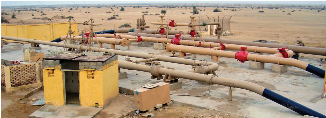
Bird eye view with MVA of Transmission Structure of Repeater Station Jhampir
