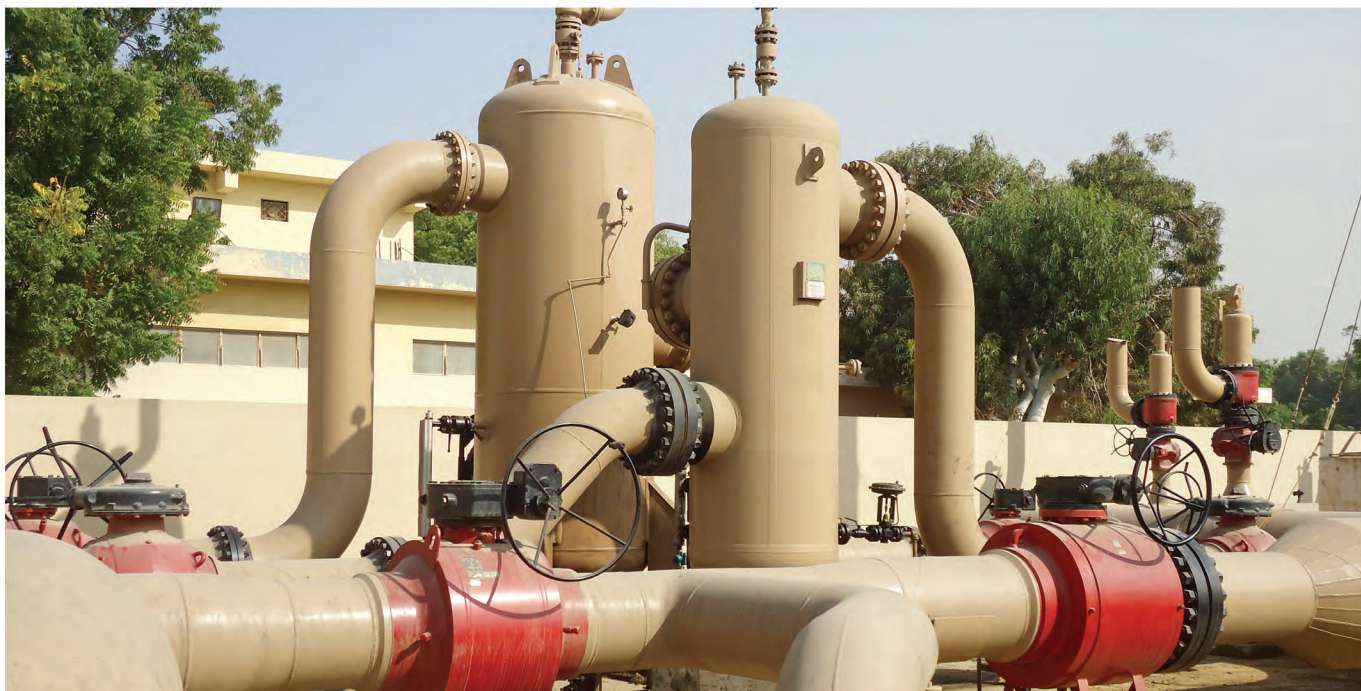
Scrubbers at SMS-II at Karachi Terminal, Section IV Transmission department
