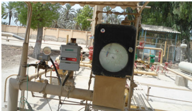
SMS Rohri, Flow Computer and Flow Recorder
