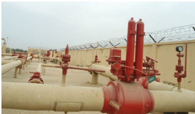
Main Valve Assembly at HQ-1
