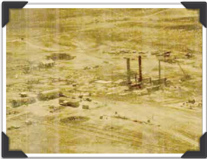
Gas Purification Plant, Early Stages
