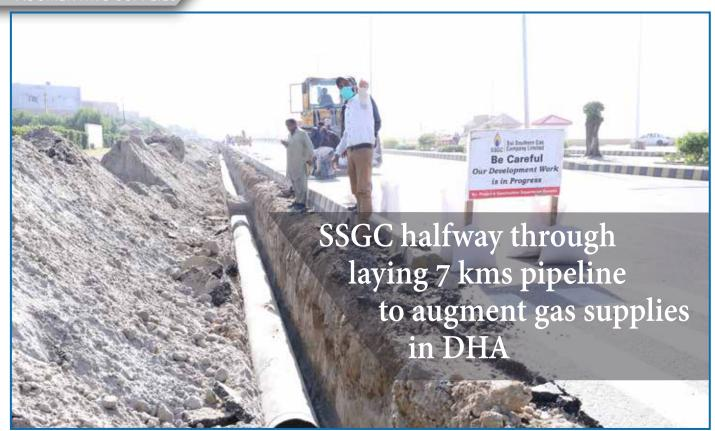
or augmenting gas supply to a number of areas in DHA and Clifton, Karachi, SSGC is working full throttle on laying a 7-km long, 20 inch diameter gas pipeline that would transport gas from the site of Dolmen Mall Clifton (DMC) to the DHA Water Desalination Plant. This 20" dia. pipeline is midway through its completion
