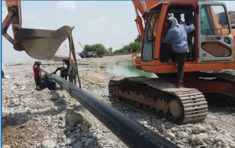
July 2020, heavy rain in Balochistan damaged the 12 dia. gas pipeline in Bibi Nani area located between the towns of Quetta and Sibi. Due to the flood situation, it took the Company's concerned technical teams more than a day to reach the location to repair the
