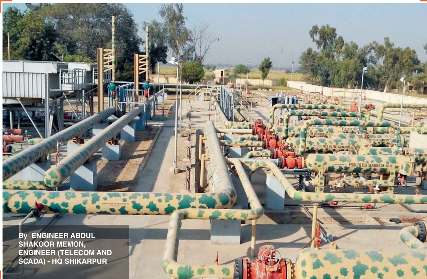
Bird's eye view of main Installation's Peco Filter Separators of Compressor at HQ Shikarpur
