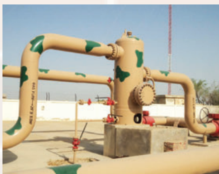
Inlet gas scrubber at HQ-2 Nawabshah
