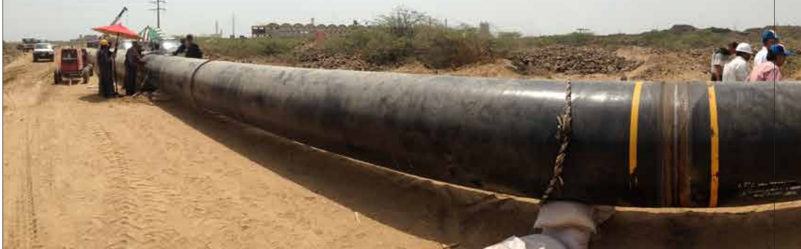
A panoramic view of the 42" dia pipeline at the site of the RLNG project at Port Qasim
