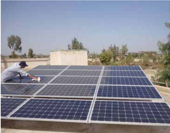
CP Solar System in HQ Dadu Section at RS Tharari Mohbat KMP 208.5. Cleaning of solar modules is in progress for better efficiency of CP solar system
