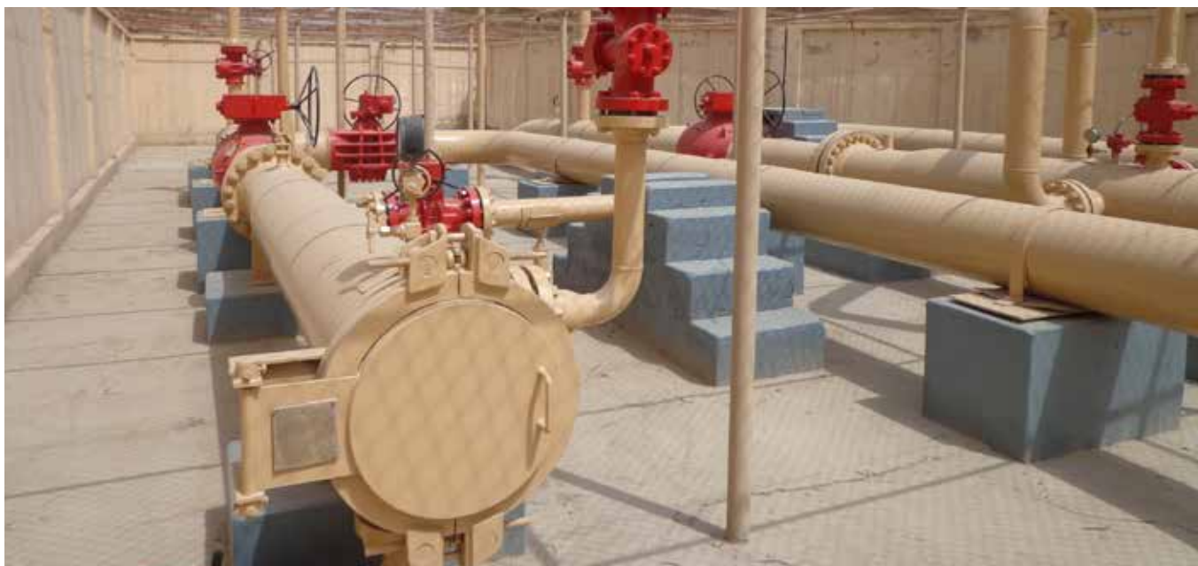
Valve assembly and PIG launching and receiving facility on 18dia and 20dia at HQ Dadu KMP 264
