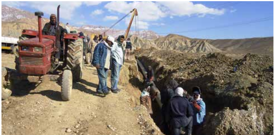
With mountains in the background, SSGC's P&C team involved in pipeline laying
