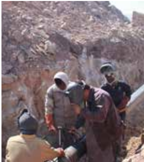
Joint weld being done on the pipeline
