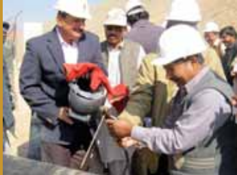
First welding - Zarghun 04
