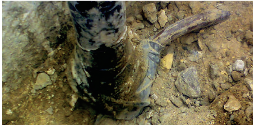
Under ground clamp that was removed by the maintenance Team
