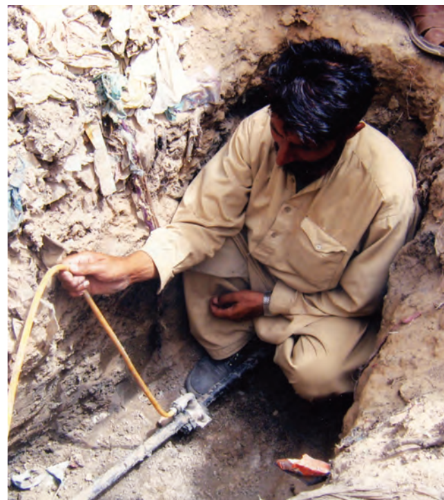
Under ground clamp that was removed by the maintenance team
