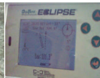
Online Tracking of Pilot Bore
