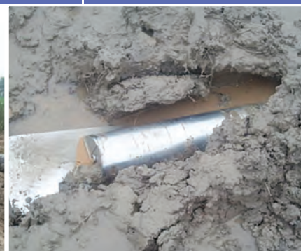
Pilot Bore completed
