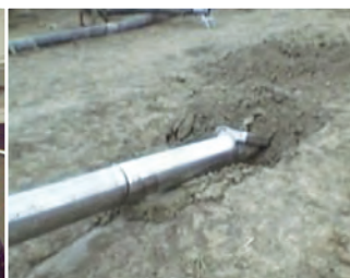
Starting the Pilot Bore
