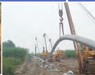
Preparing for Pipe Pulling
