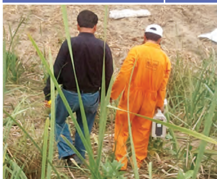
Manual Tracking of Pilot Bore by Walkover Locator
