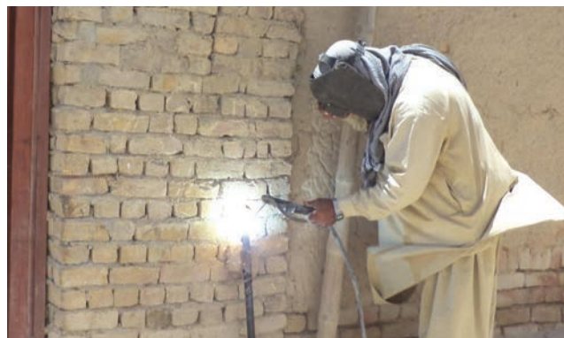
S/V being welded by the City Zone worker
