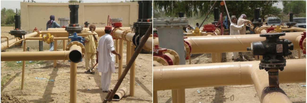
(Top to bottom) Segregation work in progress at SMS Mehrabpur
