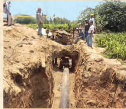
Focused: Company technicians and workers laying down 16" dia pipeline to meet Landhi Industrial Area's demand
