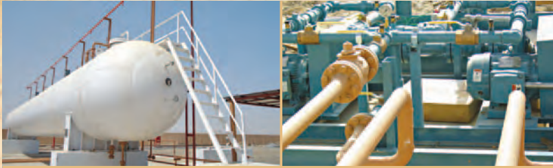
Alternative Sources: A view of the LPG Air-Mix Plant Commissioned in Noshki, Balochistan
