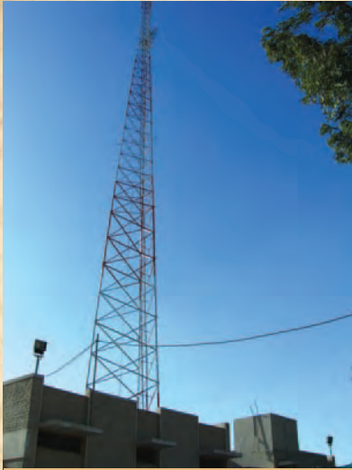
Telecommunications: A view of the Repeater Station in Tando Adam Khan
