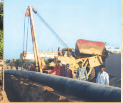
Committed: Technicians and workers laying down 24" dia supply main at National Industrial Park, Korangi Creek
