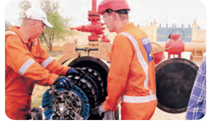
Intelligent Pigging carried out between Nawabshah HQ2 to Karachi Terminal in fine segments by SSGC and Rosen Inc. engineers.
