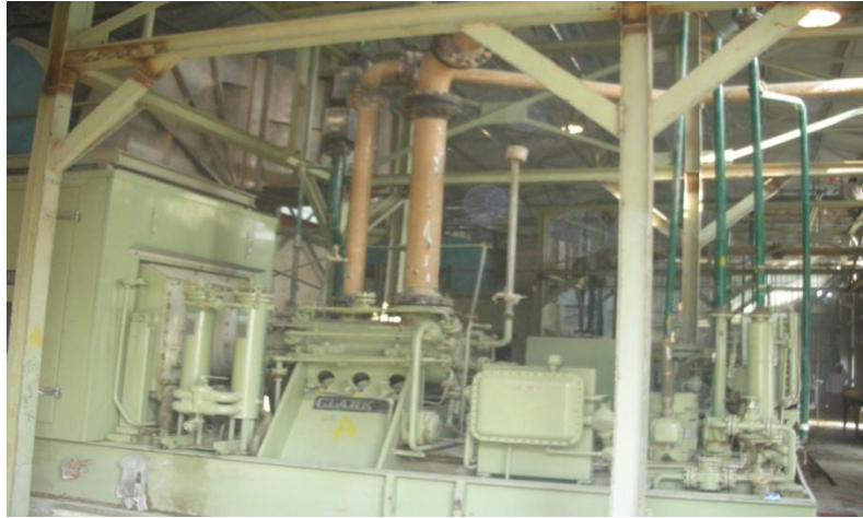
A view of turbo compressors at daur
